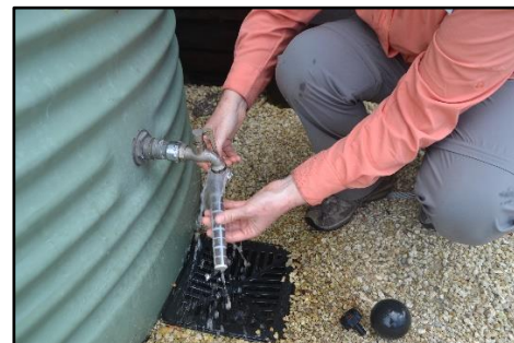
Rinse the filter; put all back together
