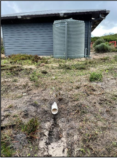
A well cleared drainage outlet
