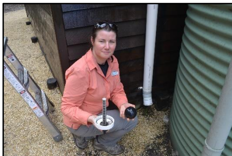
Remove the cap (with filter) and the ball valve
