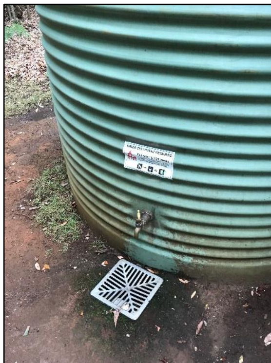
Correct location of sticker: on the tank, just above the tap
