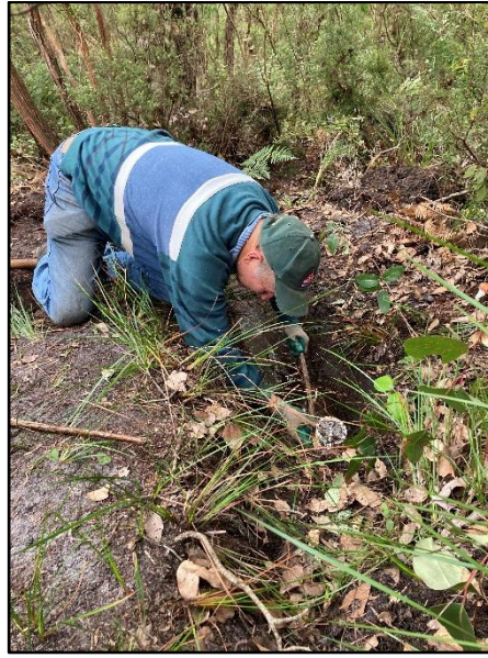
Excavating and unblocking...
